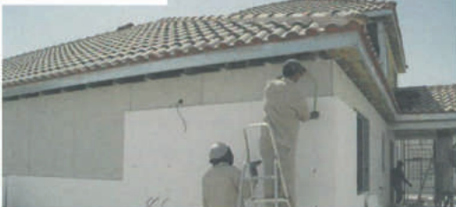
8- APPLY EXTERNAL FINISHING
