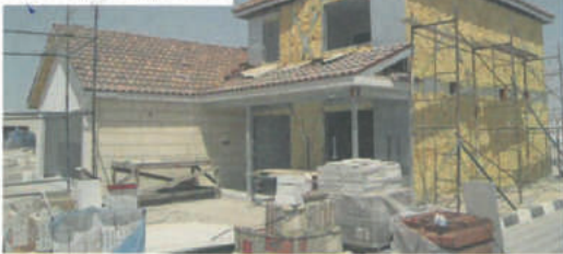
8- APPLY EXTERNAL FINISHING
